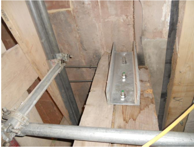
Steel support bracing to timbers in belfry.
